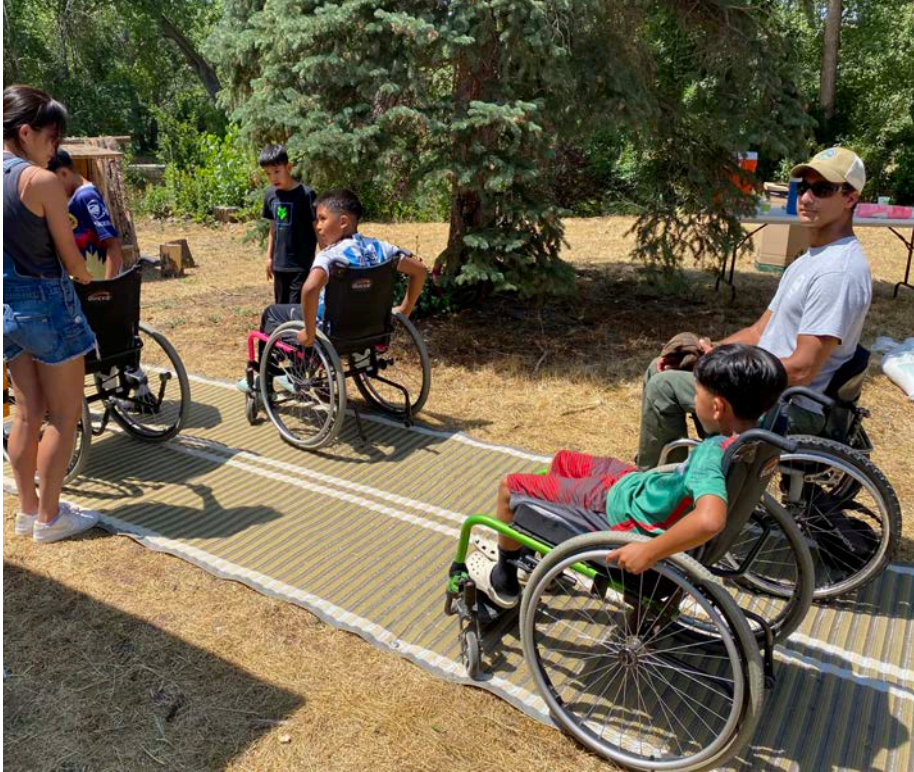
Figure 25 Mobi mats were installed in the park to improve ADA access.
