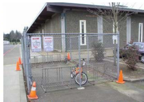
New bike parking cage along with new sidewalks and bike lanes at H.B. Lee Middle School
