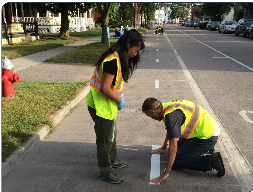
Using duct tape, these volunteers are creating a pop-up buffered bike lane in Burlington, Vermont. Photo: Street Plans Collaborative
